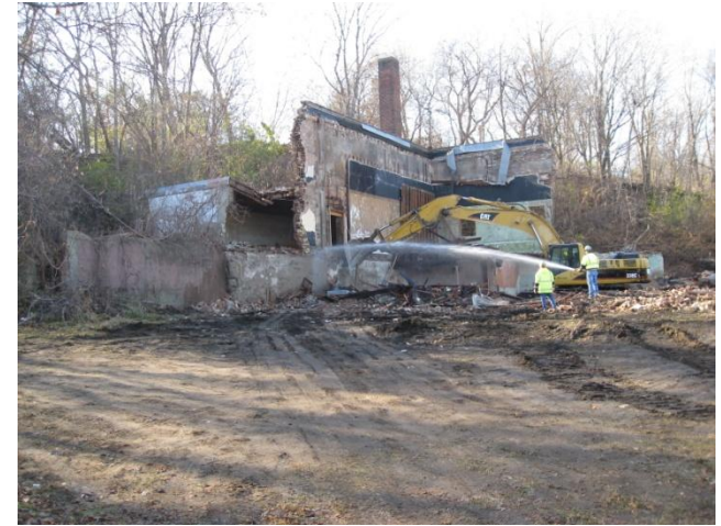
Demolition of Commercial Club
